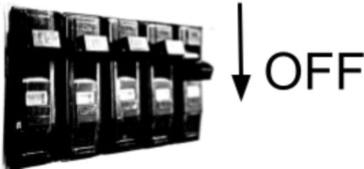
**[\*] Verify the correct breaker is off. Keep the wall switch on at your target location. When the correct breaker is off, the light will go out.**
